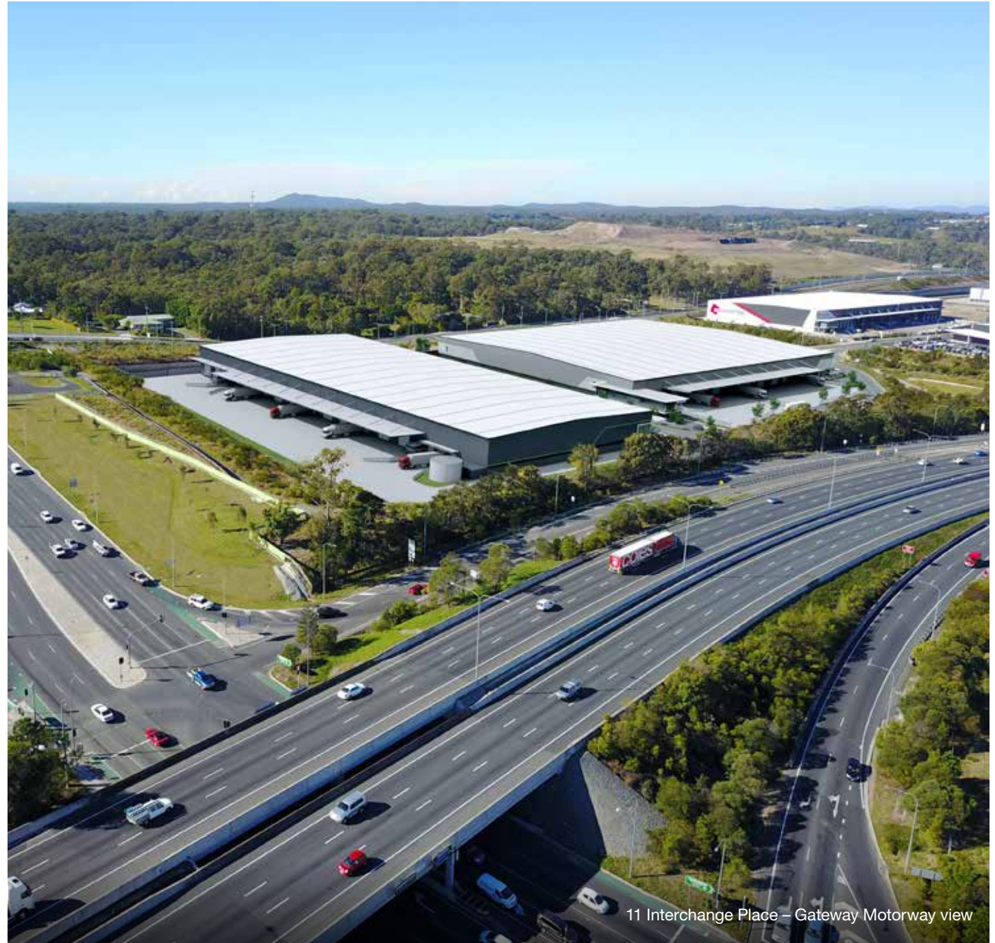
Franklyn's 8,019 sqm warehouse, showroom and national head office
