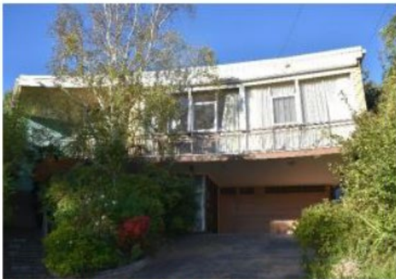
Photograph of 4 Nola Court (source: Extent Heritage Pty Ltd, 2021).
