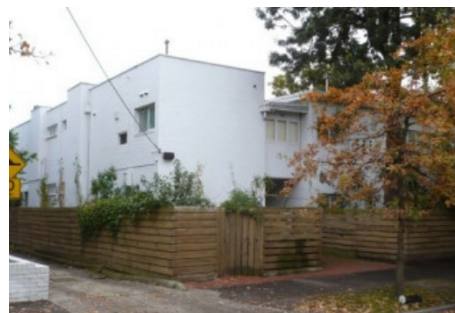
Figure 57 Clendon Flats (HO130 Armadale Precinct)
