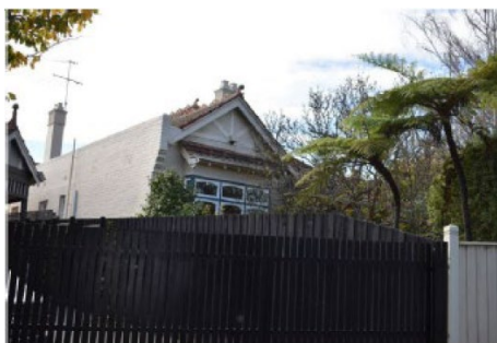
Figure 28 13 Lambert Road, Toorak
