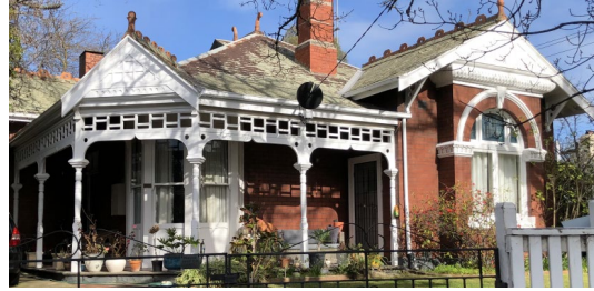
Figure 26 2 Lambert Road, Toorak
