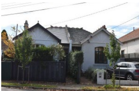
Figure 27 9 Lambert Road, Toorak
