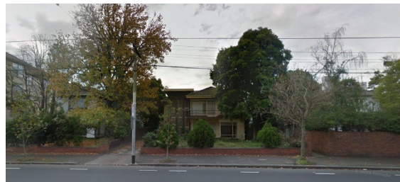
Figure 44 571 Toorak Road prior to demolition
