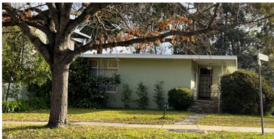
Figure 48 39 Lansell Road, Toorak - East elevation
