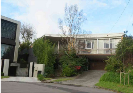
Figure 50 4 Nola Court, Toorak
