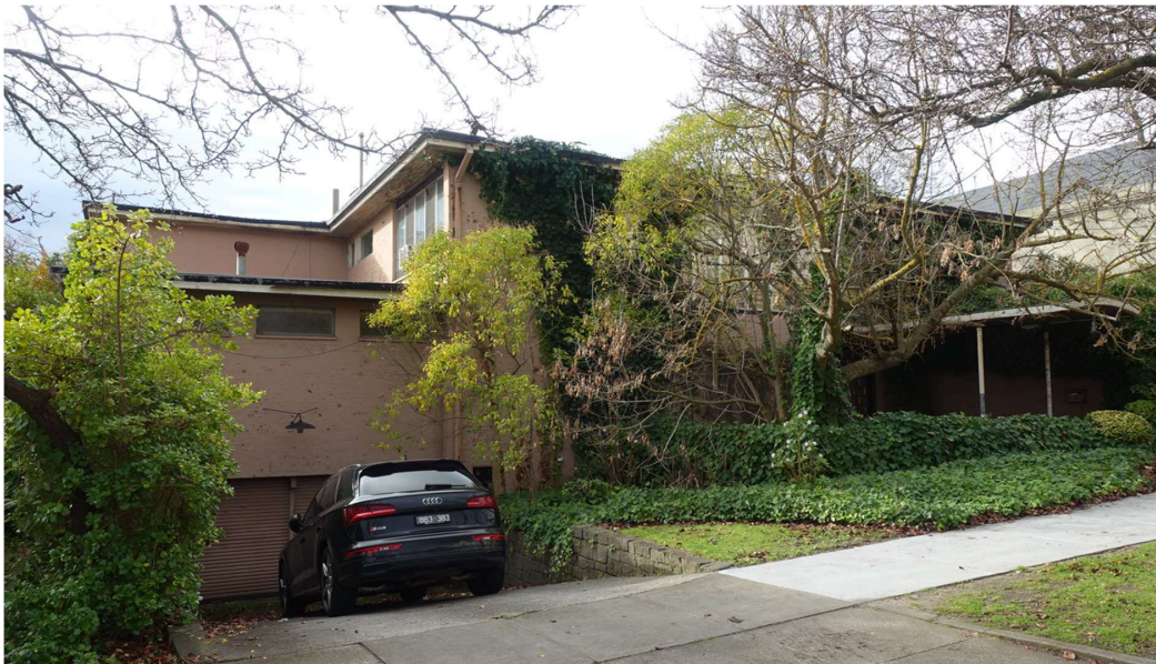
Figure 53 7 Trawalla Avenue, Toorak with 1969 addition visible above the garage
