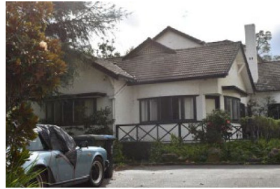
Figure 30 27 Lambert Road, Toorak
