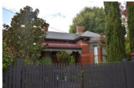
Figure 42 20 Egerton Road, Armadale 2023 view
