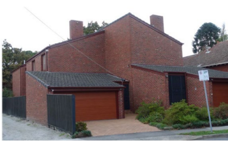
Figure 29 23 Lambert Road, Toorak
