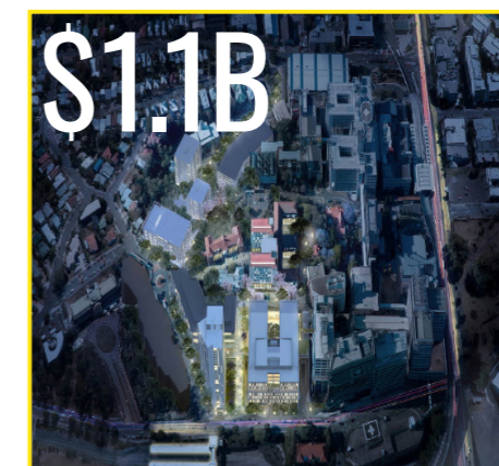
$1.1B HERSTON QUARTER HOSPITAL PRECINCT Under Construction (2020)
