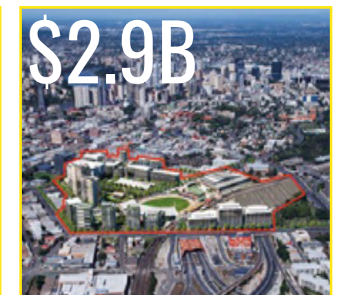
$2.9B RNA REGENERATION Under Construction (2029)
