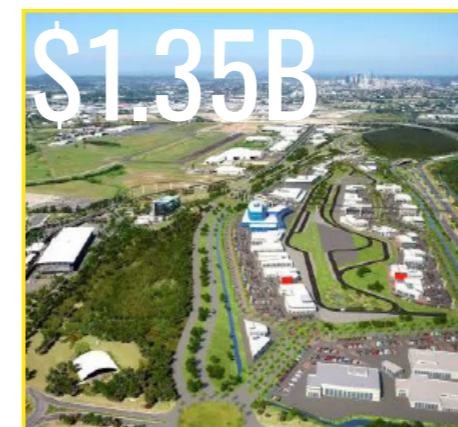
$1.35B BRISBANE AIRPORT EXPANSION Under Construction (2020)
