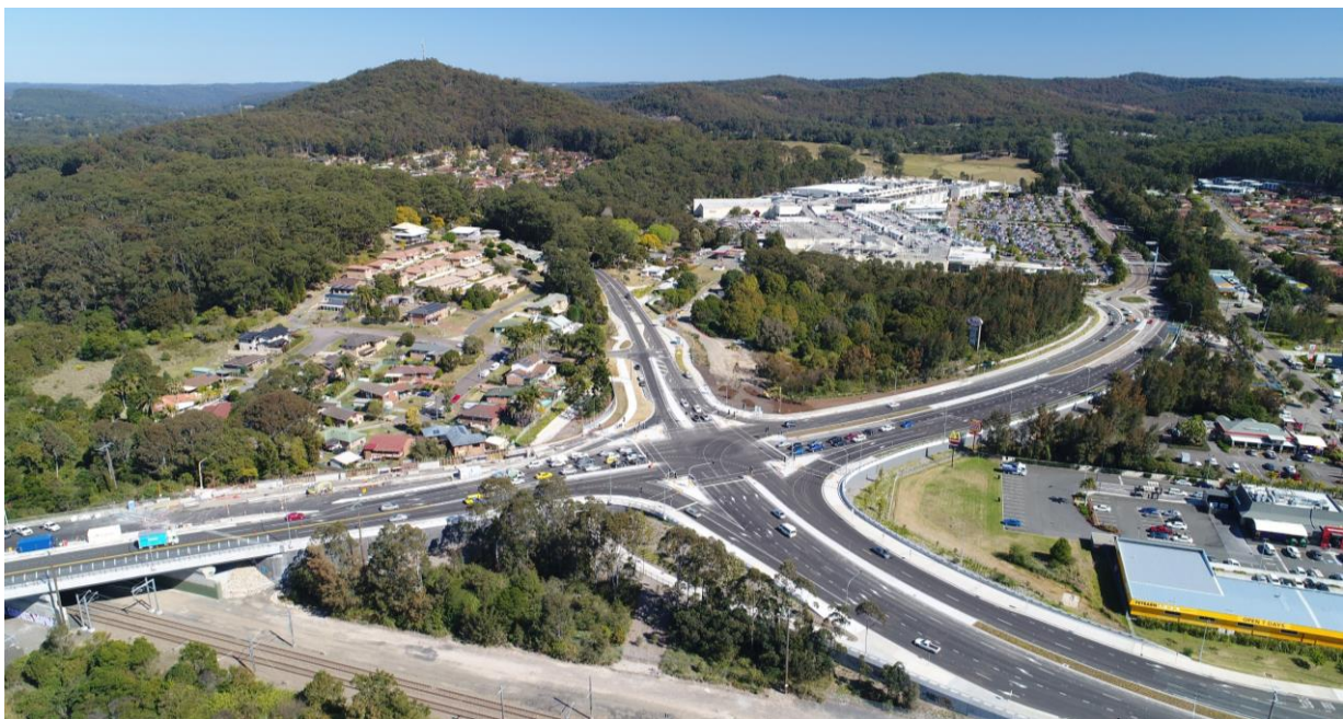
The $84 Million Pacific Hwy & Wyong Rd Tuggerah intersection upgrade is complete.
