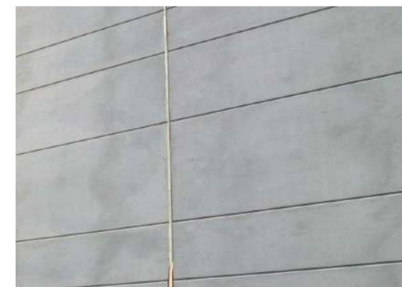
CL02 - PRE-FABRICATED EXTERNAL CLADDING PANEL WITH CONCRETE RENDER FINISH
