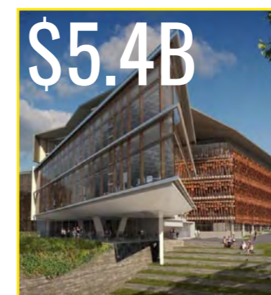
$5.4B NORTHSHORE HAMILTON Under Construction (2036)
