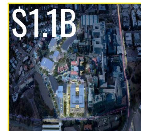
$1.1B HERSTON QUARTER HOSPITAL PRECINCT Under Construction (2020)
