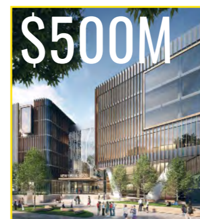
$500M SCHOOLS Under Construction (2023)
