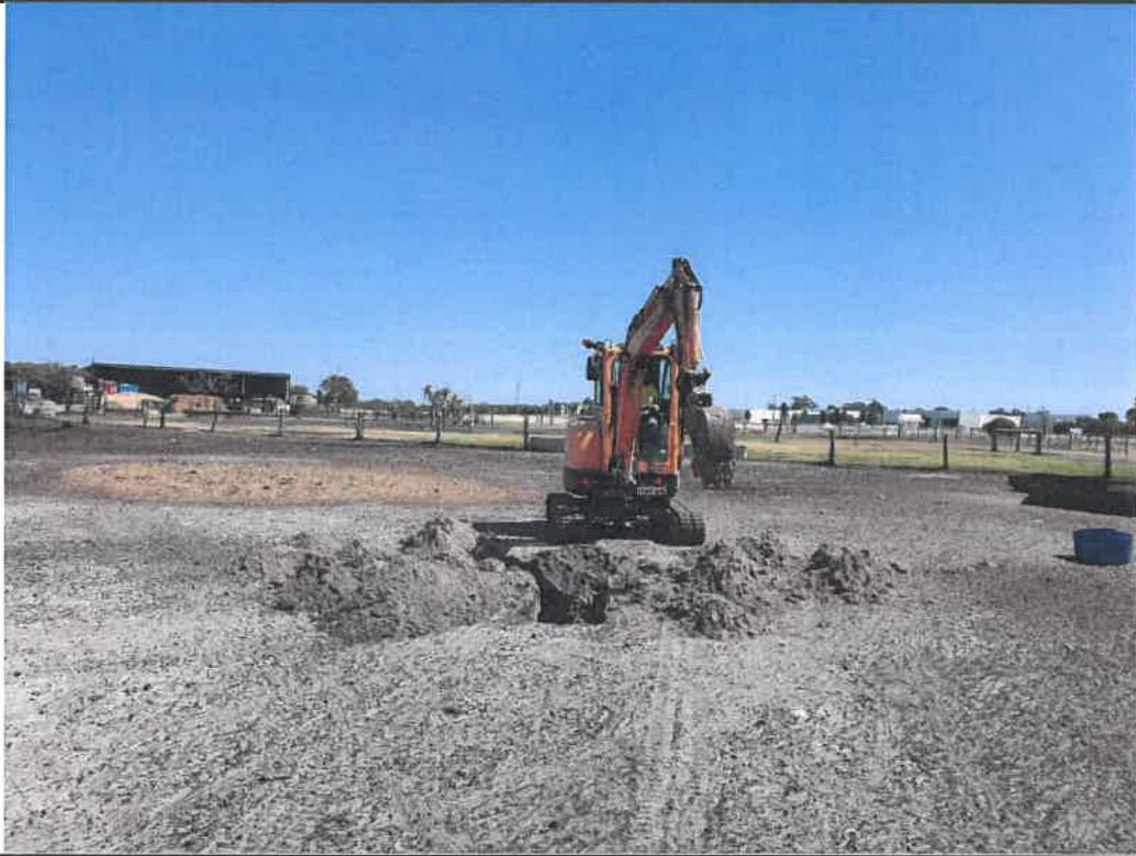
Photo 5. Test Location 04 (TH4), Sub-surface probing by an excavator
