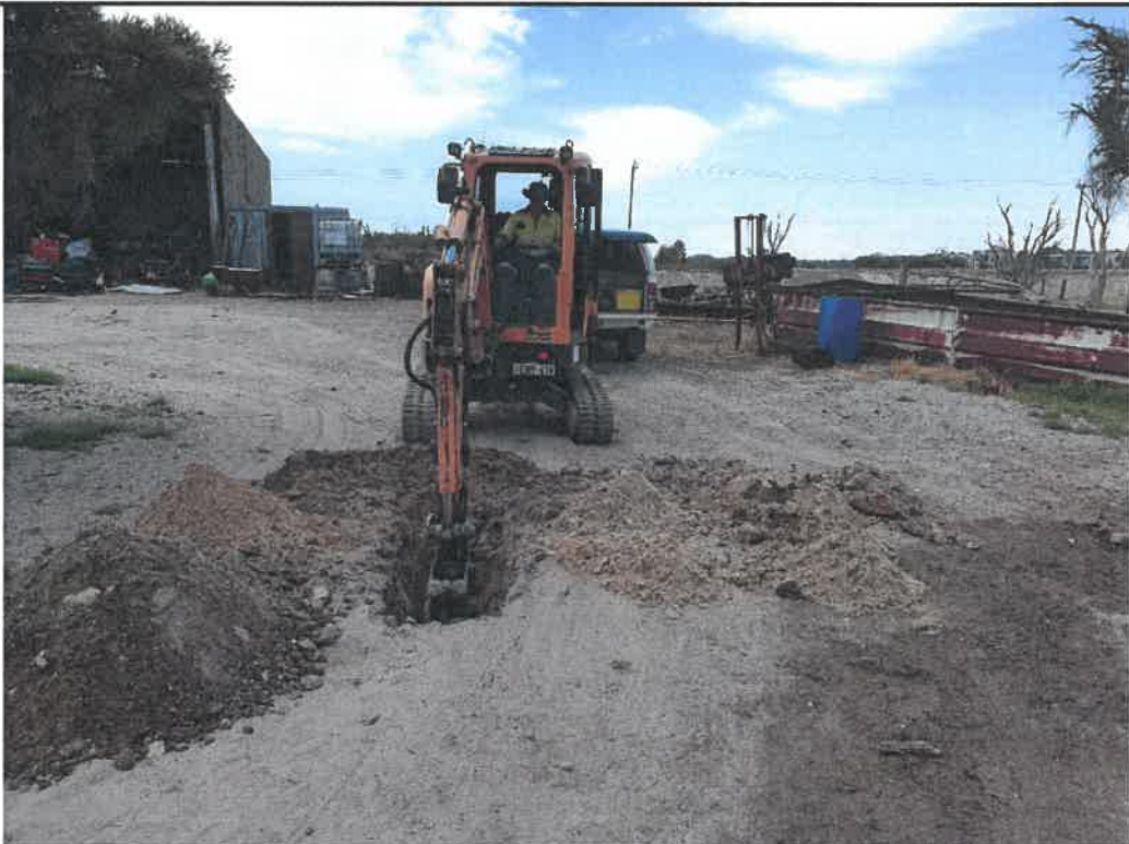
Photo 18 Test Location 15 (DCP15), Sub-surface probing by an excavator
