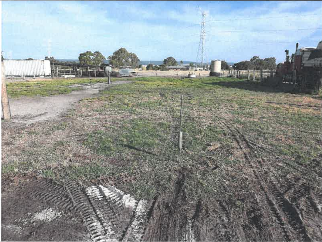
Photo 21. Test Location 19 (DCP19), Testing by a Dynamic Cone Penetrometer
