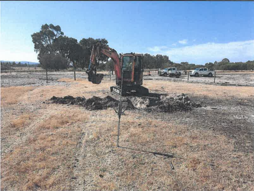
Photo 2 Test Location 01 (DCP1), Testing by a Dynamic Cone Penetrometer
