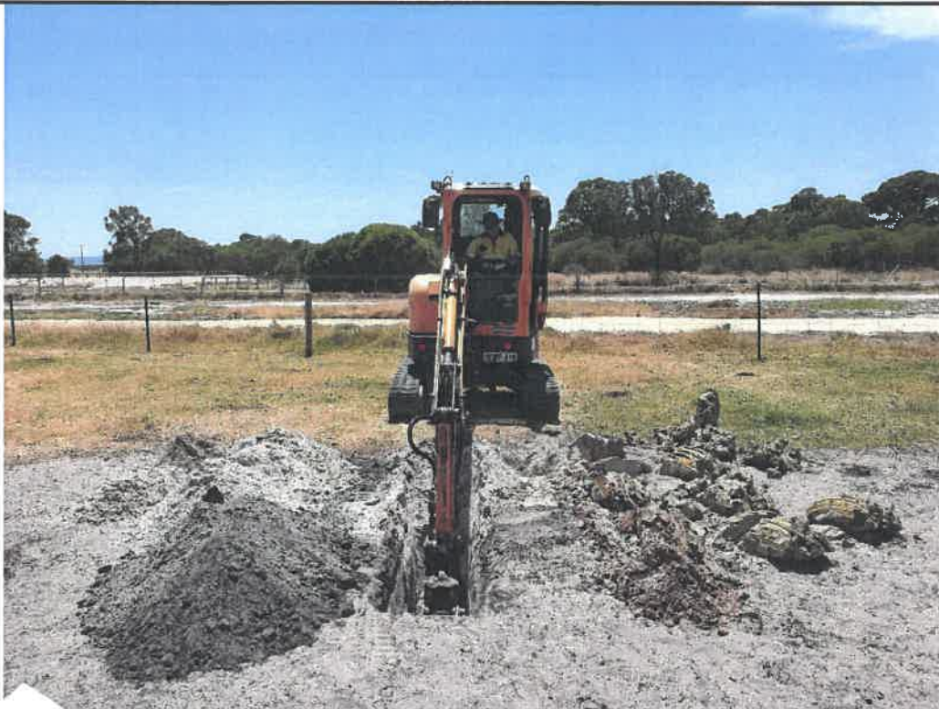
Photo 9. Test Location 07 (TH7), Sub-surface probing by an excavator
