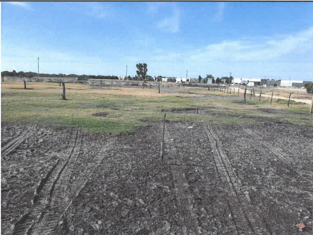
Photo 10 Test Location 08 (DCP8), Testing by a Dynamic Cone Penetrometer
