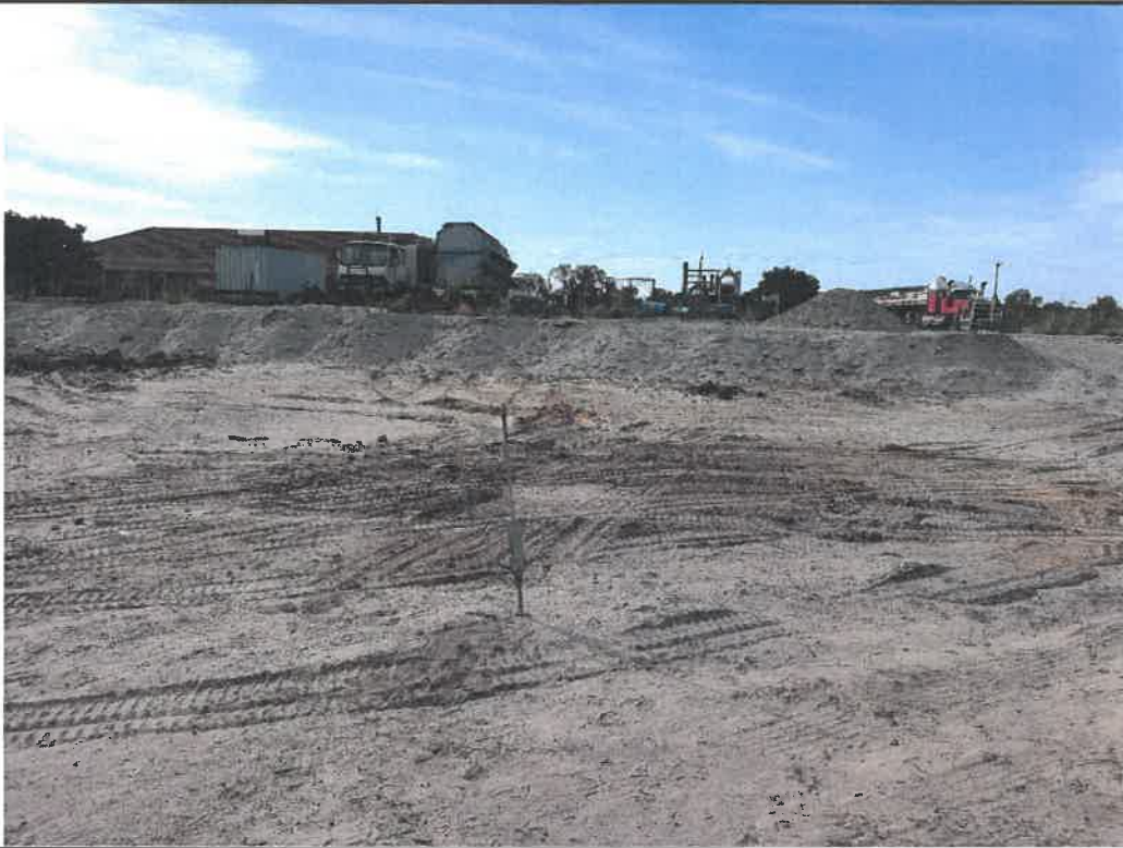
Photo 7. Test Location 05 (DCP5), Testing by a Dynamic Cone Penetrometer
