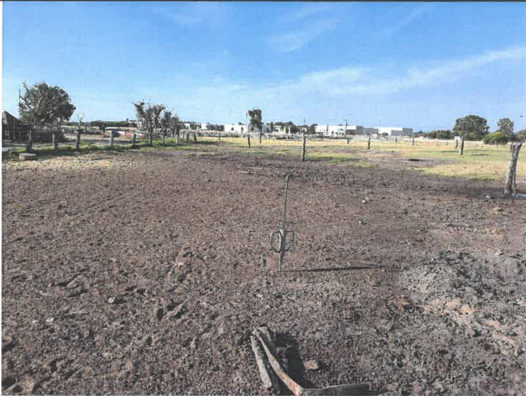
Photo 13. Test Location 11 (DCP11), Testing by a Dynamic Cone Penetrometer
