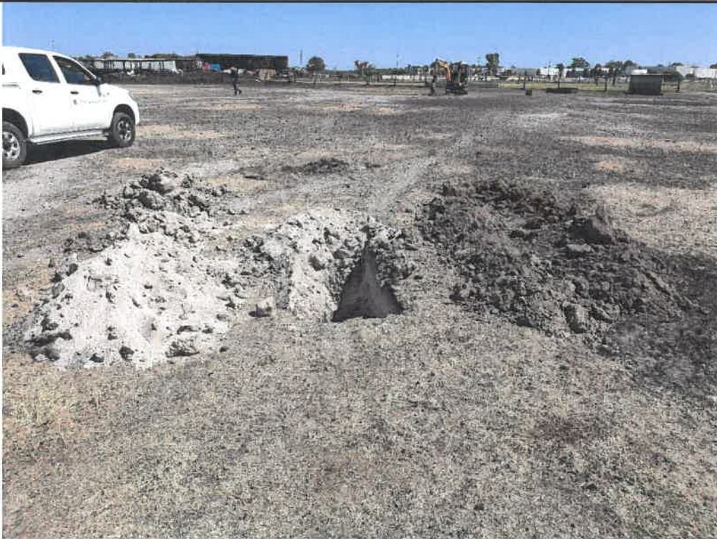
Photo 4. Soil from Test Location 03 (TH3)
