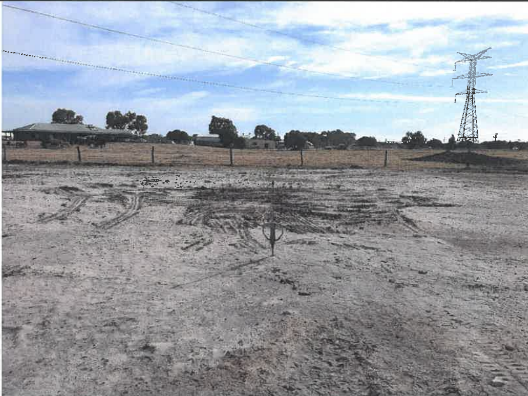
Photo 8. Test Location 06 (DCP6), Testing by a Dynamic Cone Penetrometer
