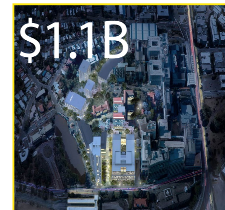
$1.1B HERSTON QUARTER HOSPITAL PRECINCT Under Construction (2020)
