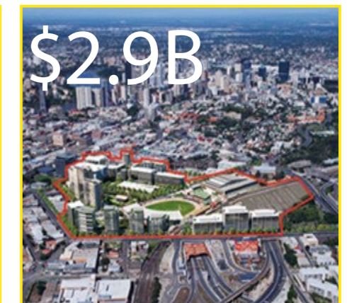
$2.9B RNA REGENERATION Under Construction (2029)
