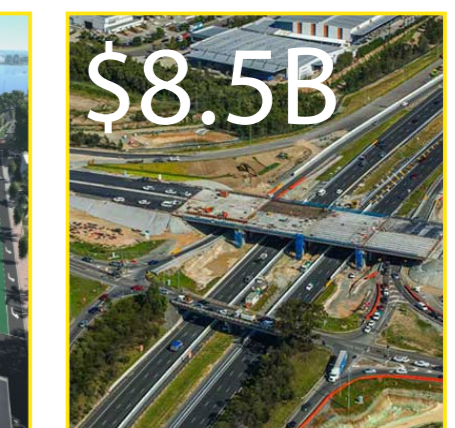
$8.5B BRUCE HIGHWAY UPGRADE Under Construction (2023)
