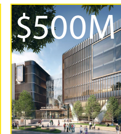
$500M SCHOOLS Under Construction (2023)
