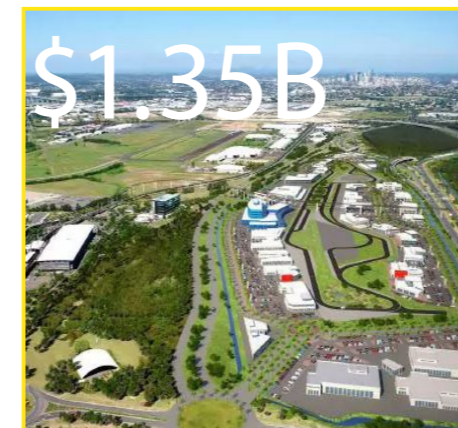
$1.35B BRISBANE AIRPORT EXPANSION Under Construction (2020)
