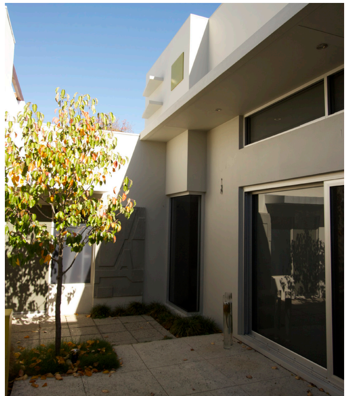
A combination of eaves and trees can provide shading to external paving and reduce the reflected heat load
