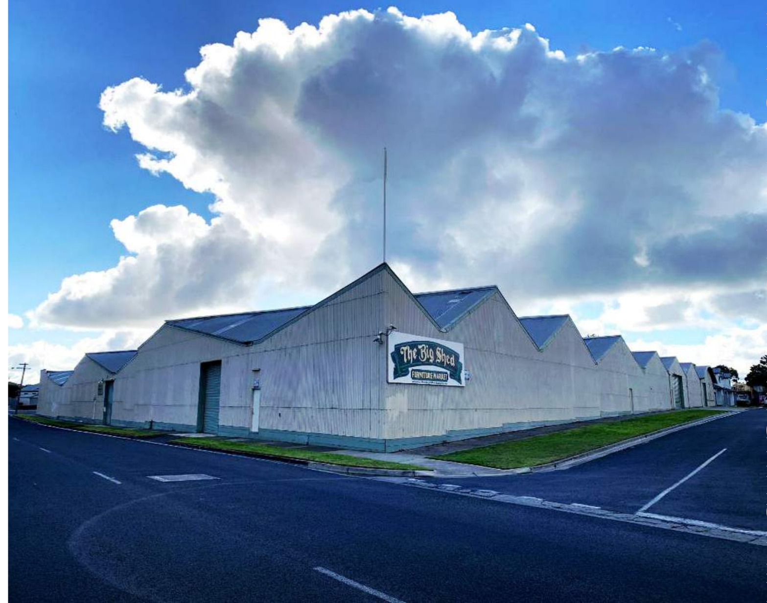
Figure 41. Previous view of the Big shed redevelopment at 135 Fitzroy Street
