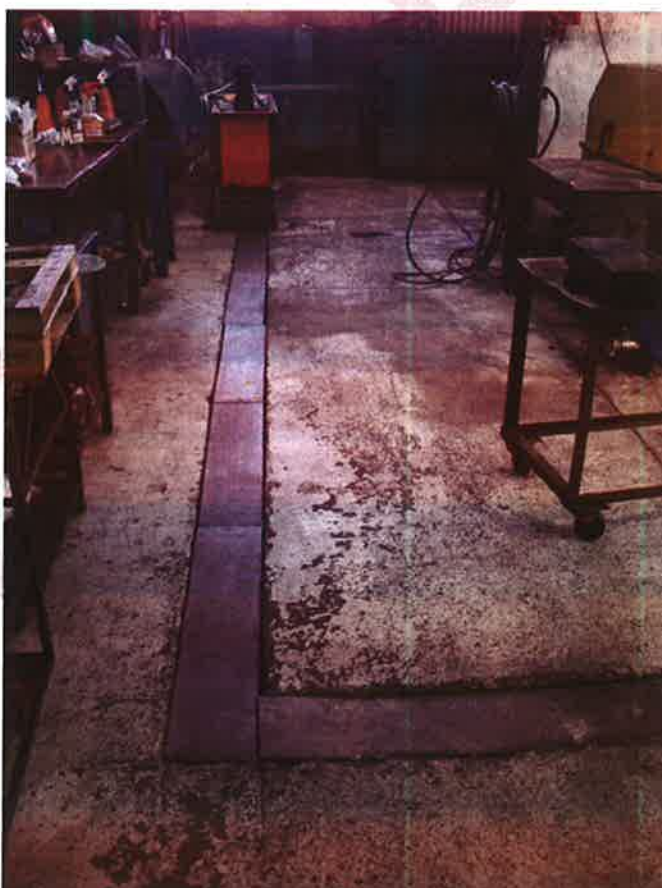
PLATE 6: Drains (leading to settling tanks) surrounding the wash down area within the workshop.
