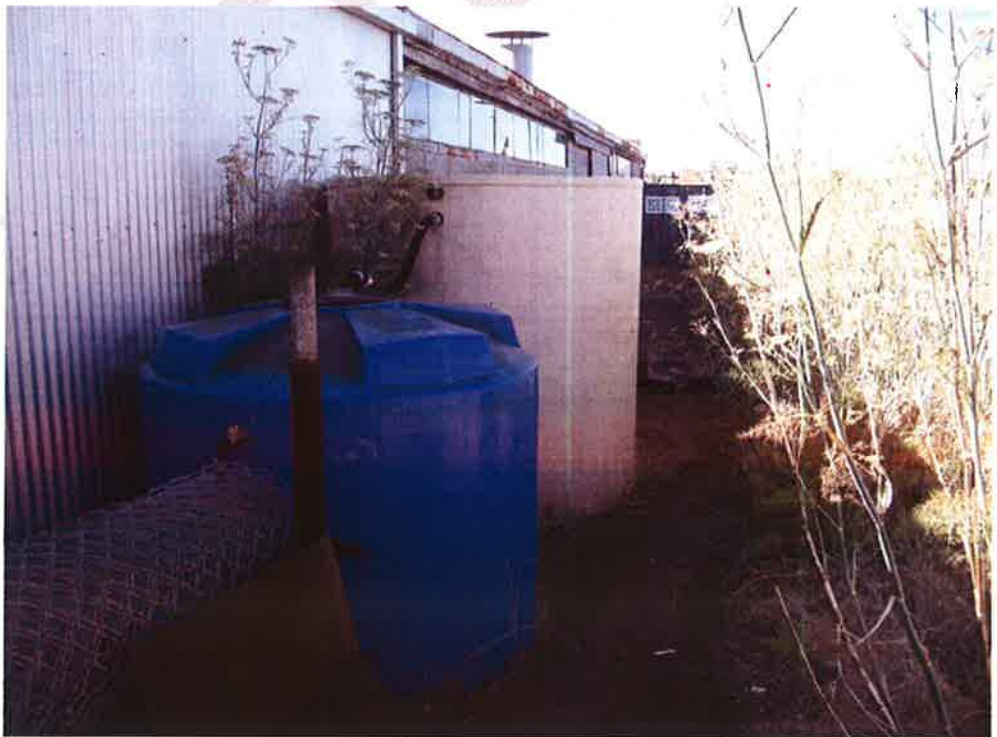
PLATE 2: Two separator tanks on the western side of the building.
