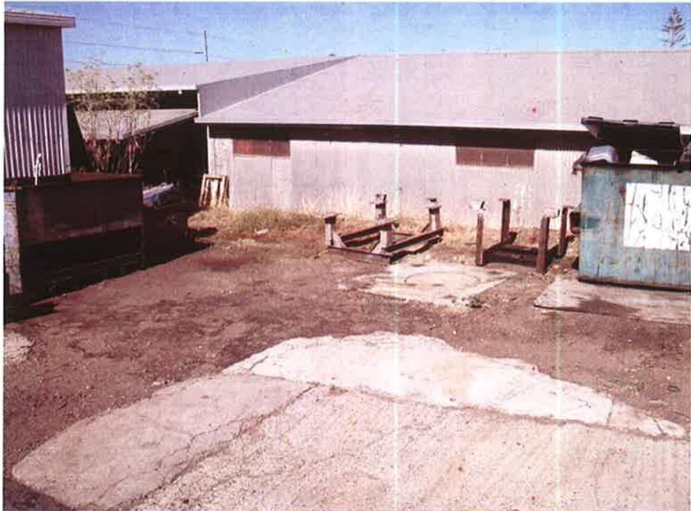
PLATE 1: Bitumen driveway at rear of property and drainage sump, visible in middle ground.
