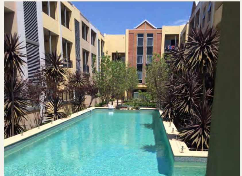
Well planted, attractive communal open space for residents and workers to recreate
