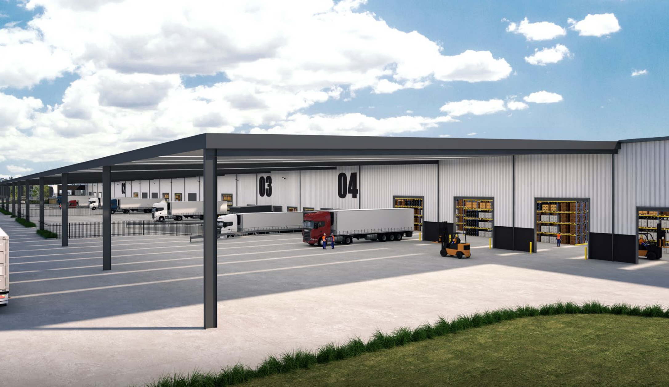
Hardstand view - Gateway@Green Road
