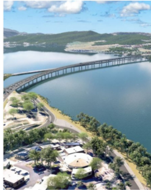
New Bridgewater Bridge – Transport Services
