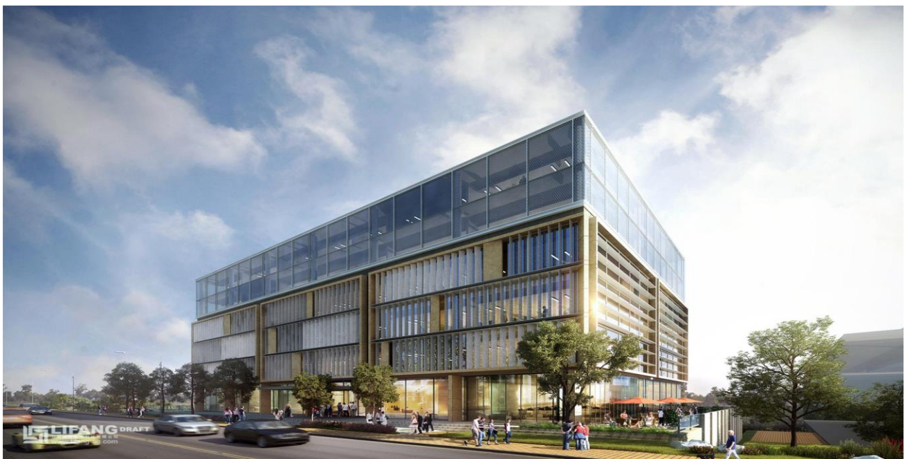
Department of Finance Building - Gosford
