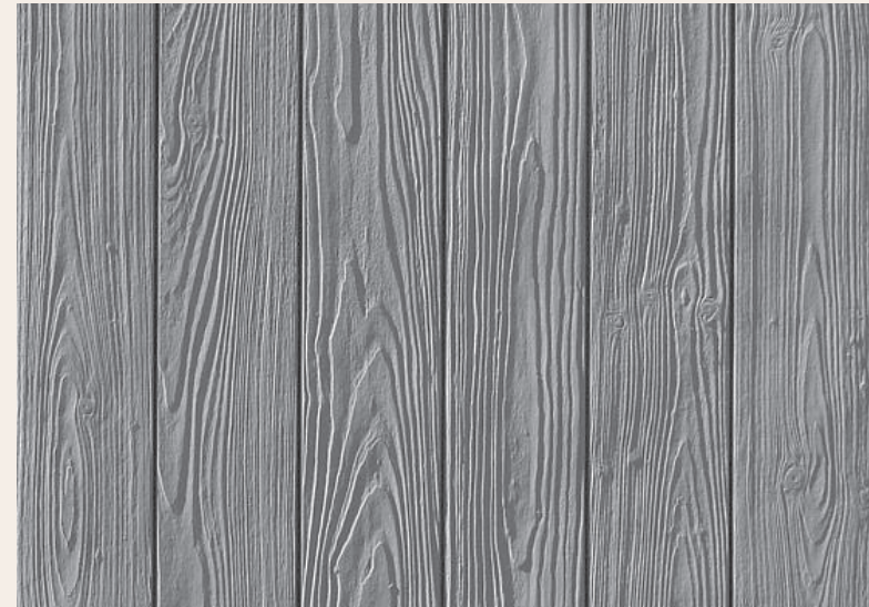
TILT PANEL DETAIL CONCRETE WALLS Engineered Facade Walls. 150mm Thick / Plain Concrete with Surf Mist whites and Concrete greys with seal coat 3 coat paint system tilt panel sand grit paint
