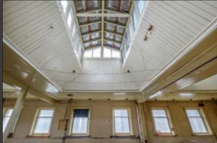
Existing top floor
