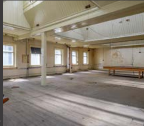
Existing top floor
