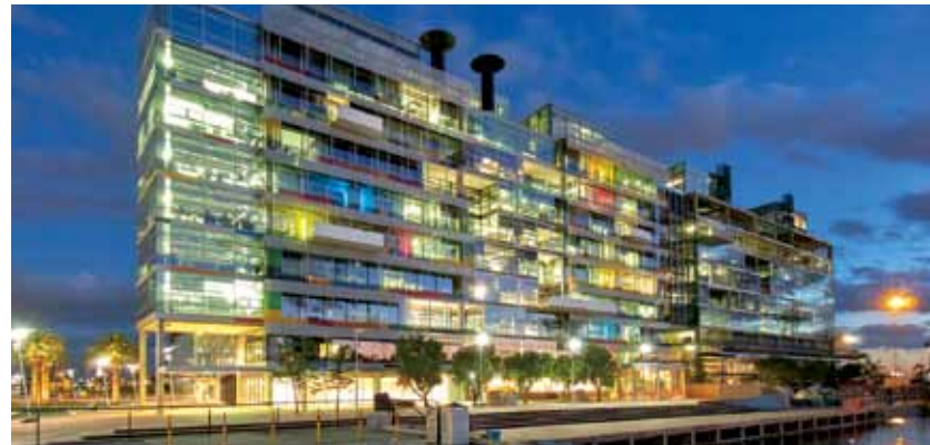
Melbourne Docklands 'Greenfield', for the National Australia Bank
