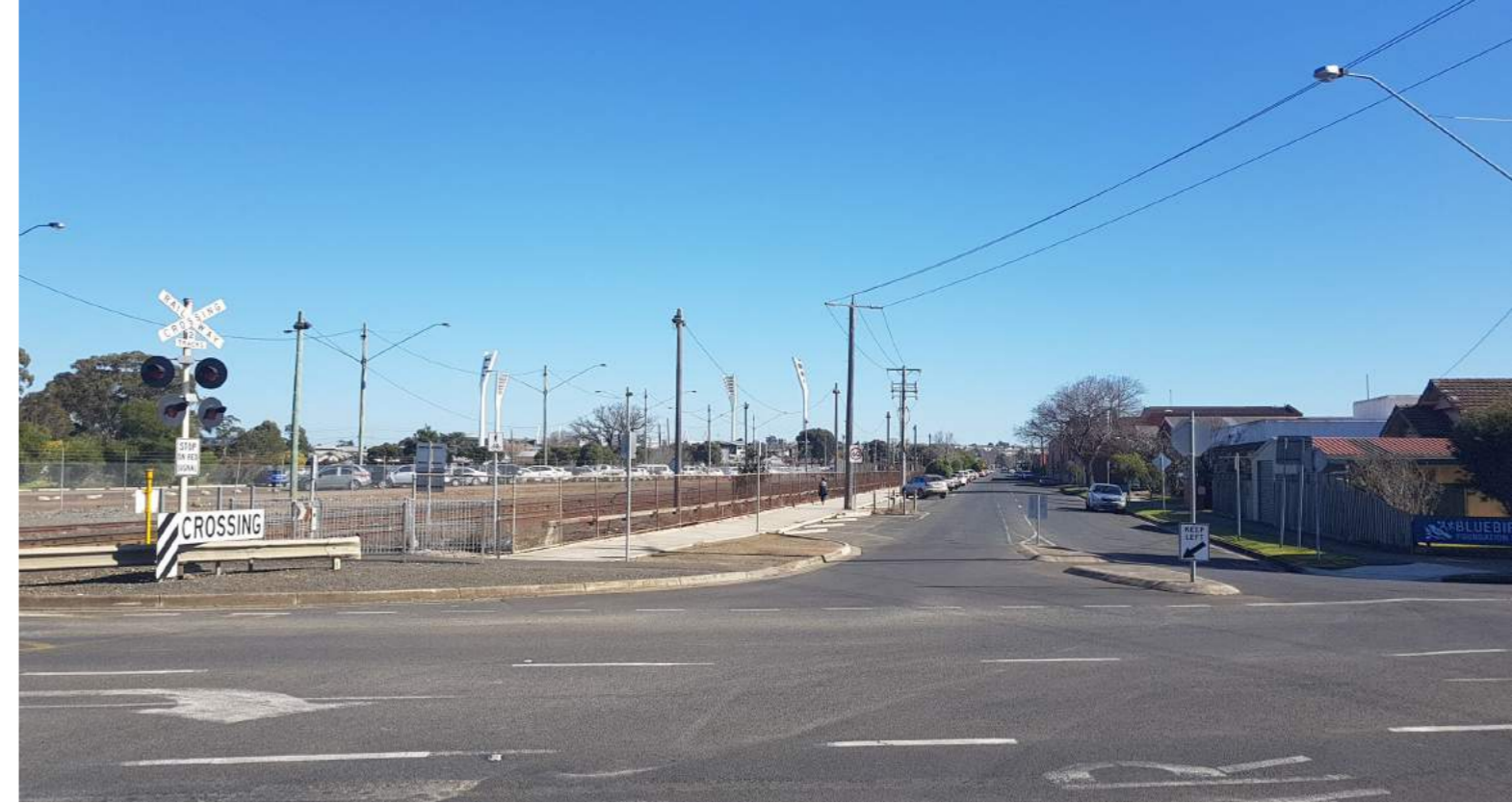
Figure 62. Existing Station Precinct, prior to removal of Barwon Water Buildings
