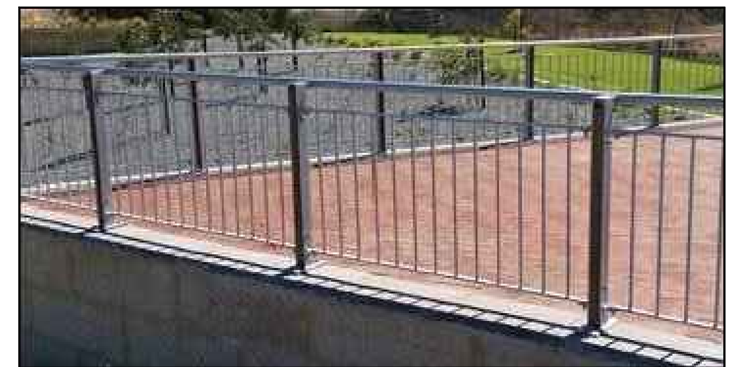
BARRIER WALL PHOTO NTS
