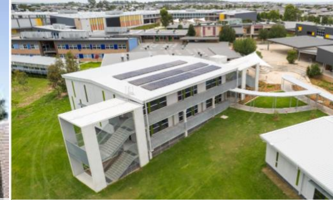
16 New Class rooms Recently Built 2024
