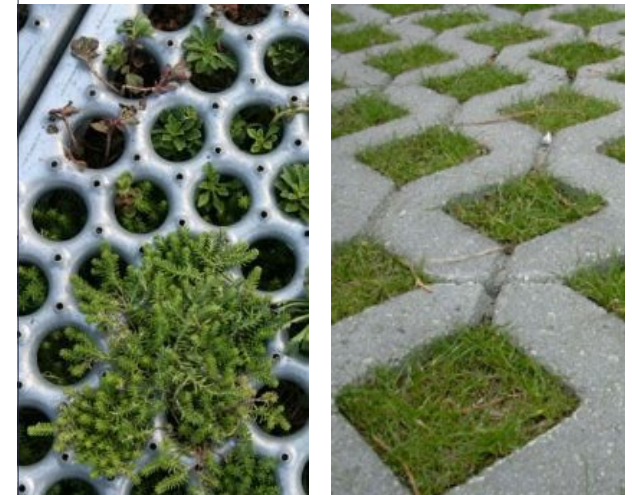
Permeable paving allows drainage to groundwater.
