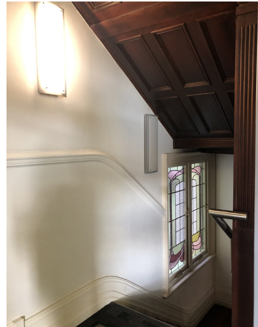
EXISTING LIGHTING TO REPLACE
