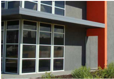
Balance natural light, whilst minimising thermal heat gain through awnings and blade walls.
