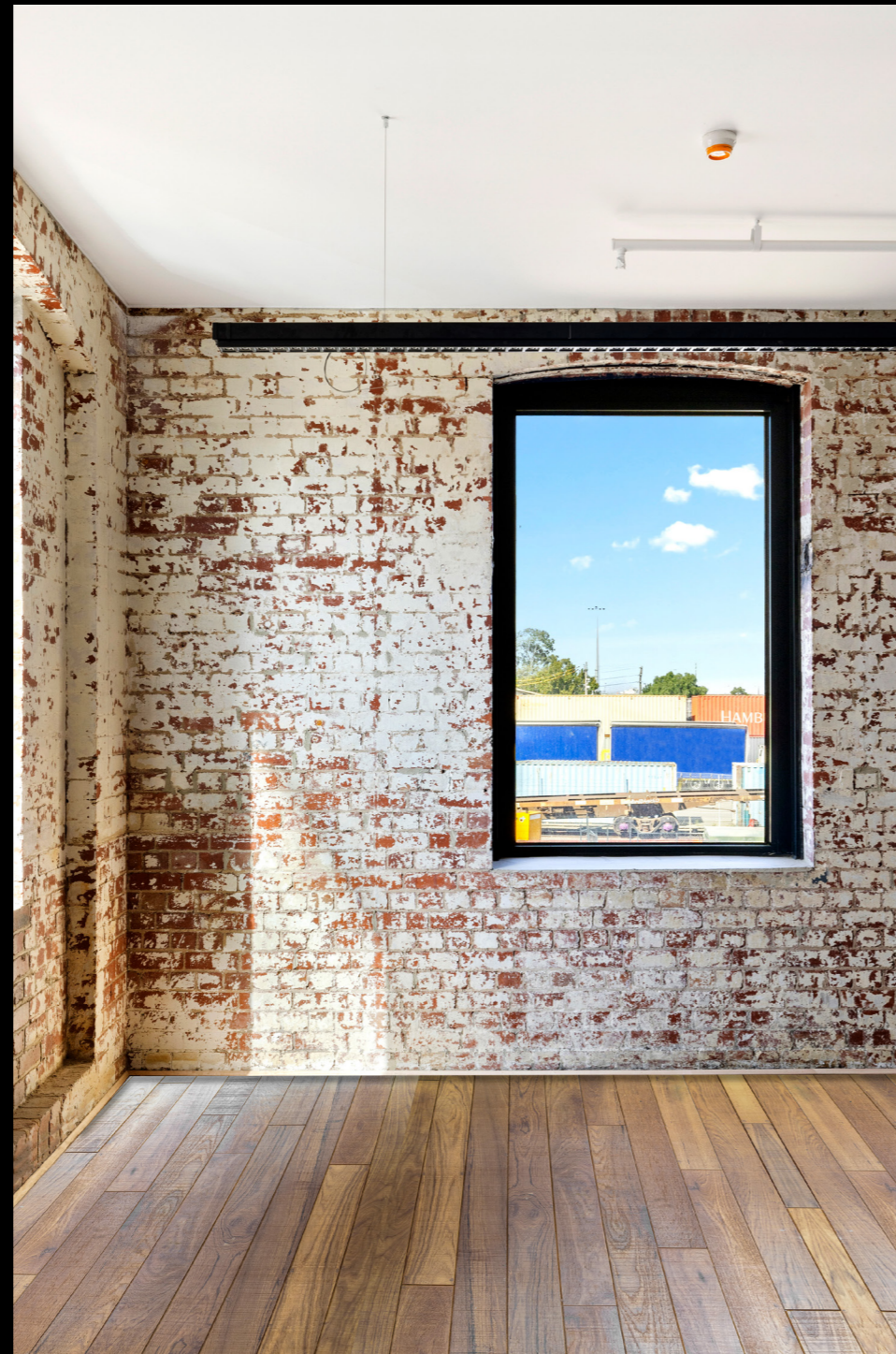
"Under construction, image at April 2023"
