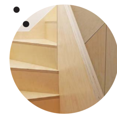
PLY WOOD STAIRCASE DESIGN WITH VOID
